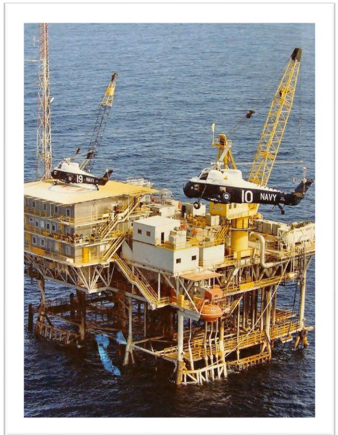
Wessex operating on the Bass Strait oil platform ‘Marlin’ during 1983. Aircraft only landed on the pad of an installation to collect personnel and material following exercises.
